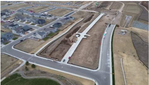
Earthwork and Paving
