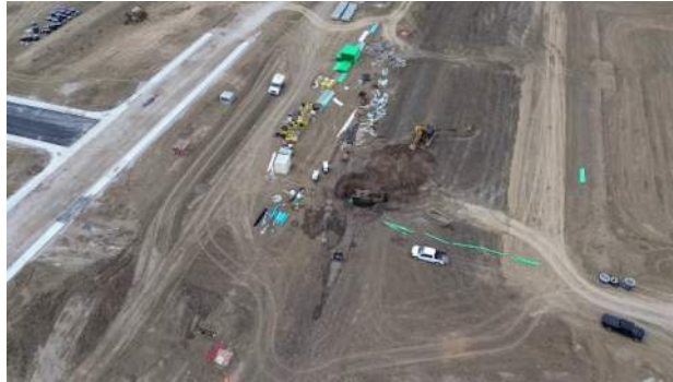
Sanitary Sewer Installation
