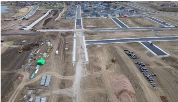
Colorado River Drive
