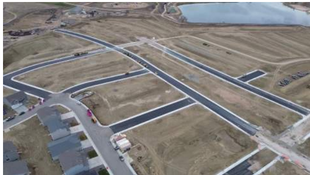
Northwest Section of Site
